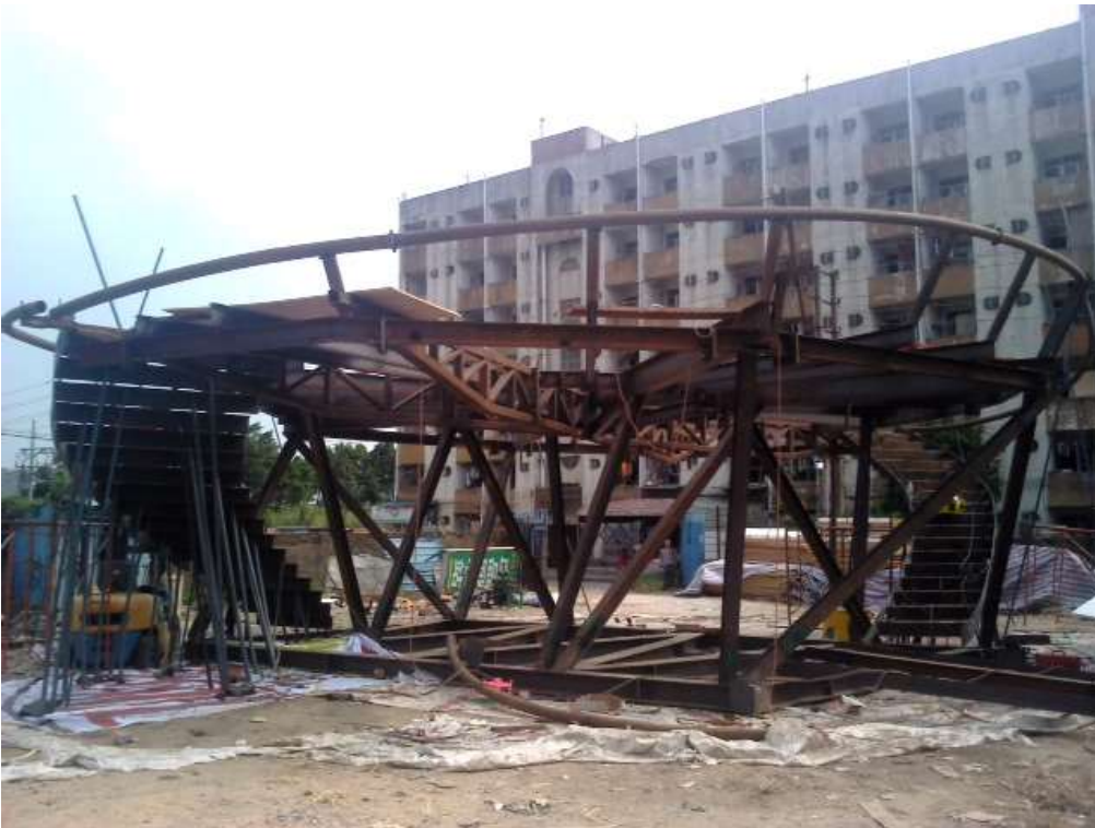
Figure 13 – ‘Dry run’ of construction of base structure
