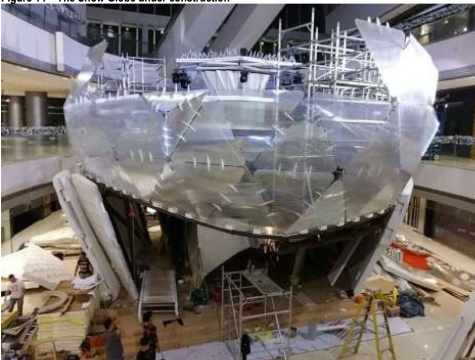
Figure 14 – The Snow Globe under construction
