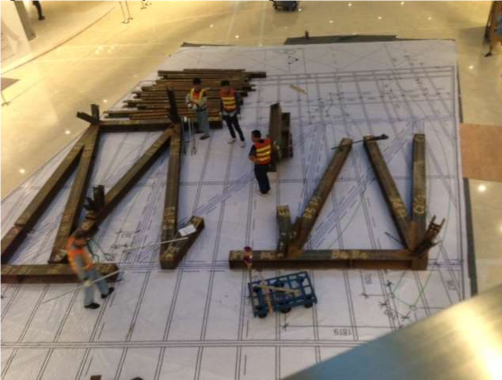
Figure 12 – Fabrication directly over the 1:1 scale drawings
