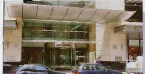
60 Castlereagh Street, Sydney NSW (Glass Feature Walls)
