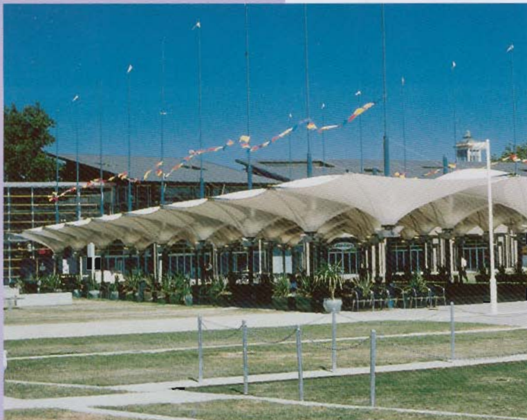
Citation Special Applications Shade Structures Pacific Pty Ltd -Fox Studios Parade Ring, Sydney NSW (Inverted Cones/Collapsible Demountable)
