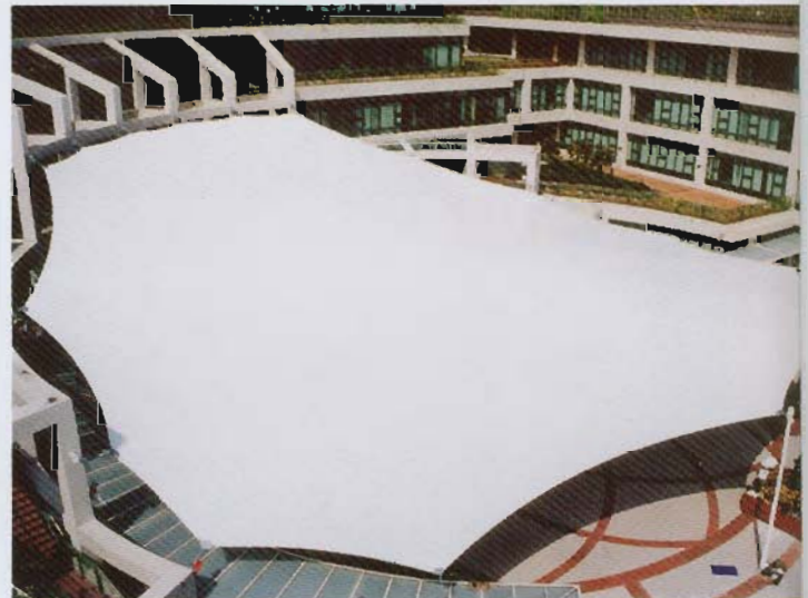
Citation Special Applications Structurflex Limited -Hong Kong Institute of Education Tai Po, N.T. Hong Kong (Removable Canopy)
