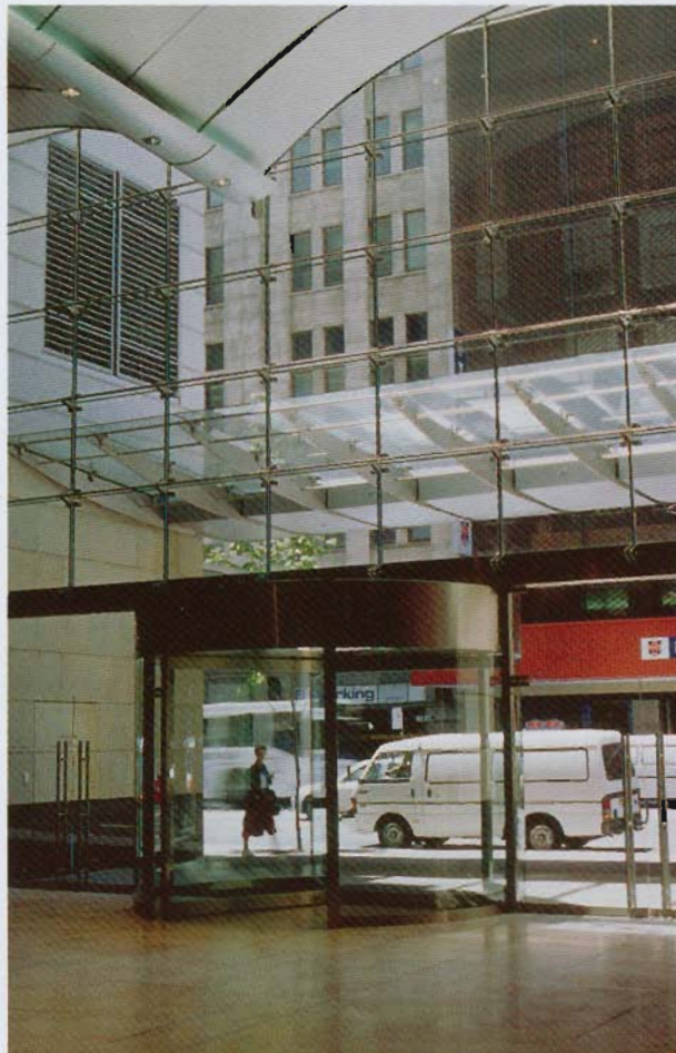
Winner Small Structures Connell Wagner Pty Ltd - 60 Castlereagh Street, Sydney NSW (Glass Feature Walls)
