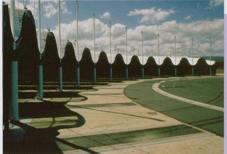
Citation Small Structures Morris-Nunn & Associates Pty Ltd -Inveresk Round House, Inveresk Railyards Launceston TAS
