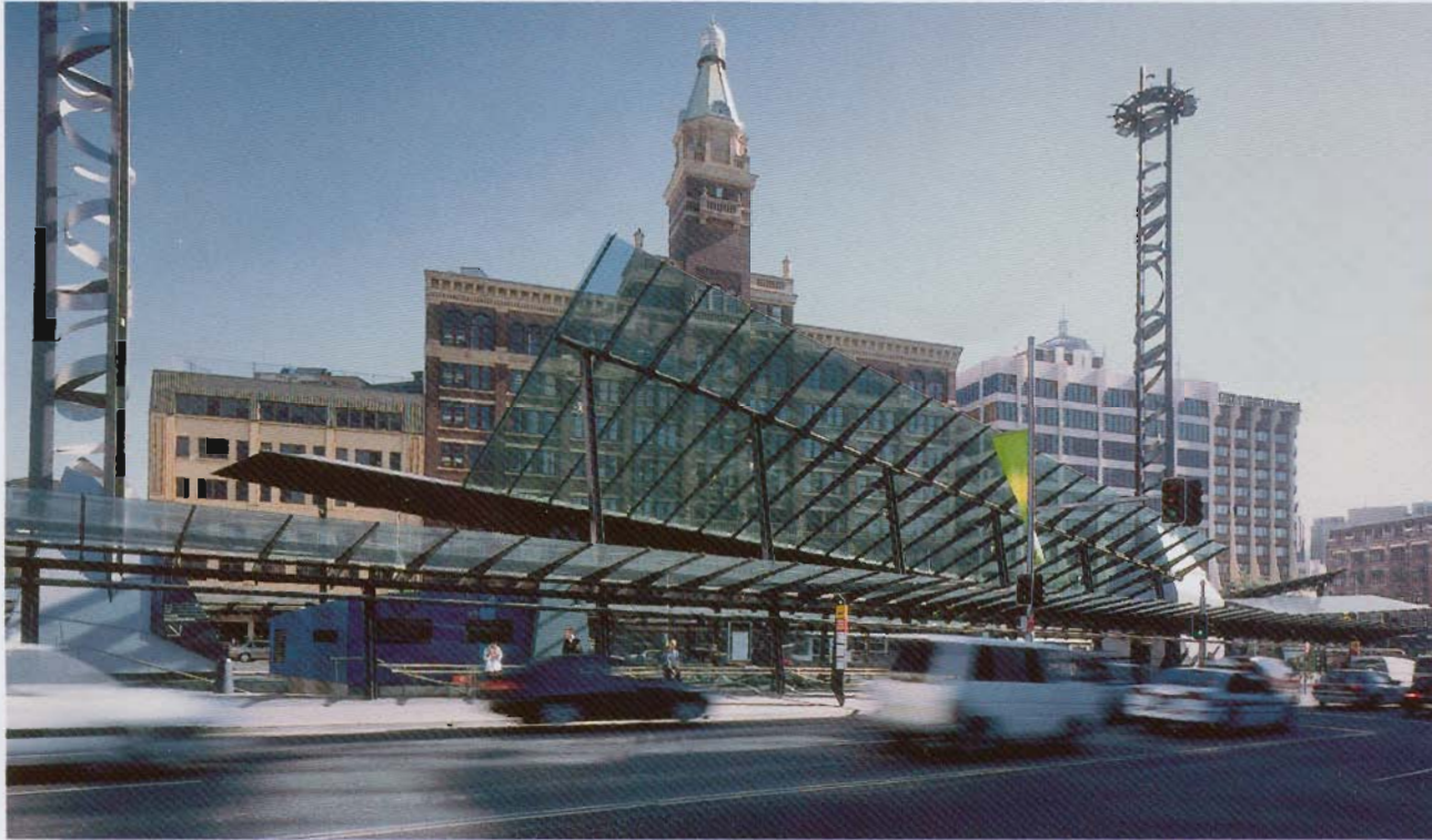
Winner Large Structures Connell Wagner Pty Ltd - Railway Square, Sydney NSW (Glazed Canopies)
