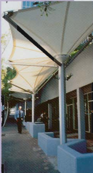
Zenith Centre NSW (Canopy)
