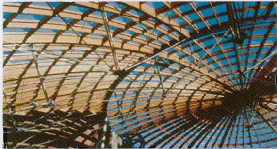
Forestry Tasmania Headquarters, Hobart TAS
