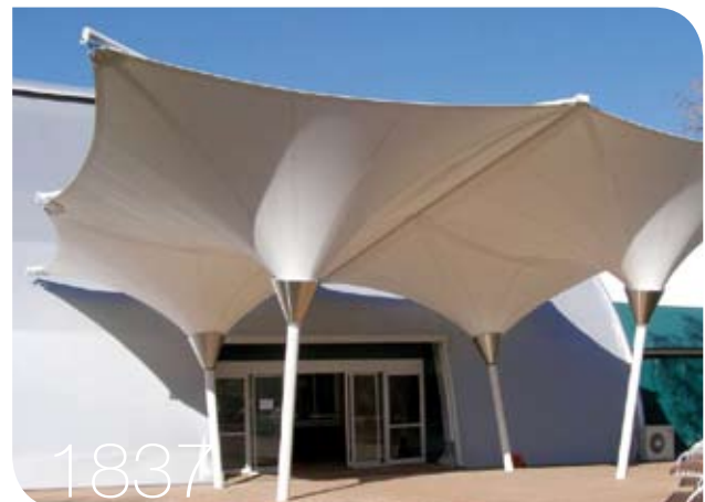
Mpowerdome Entry Structure
