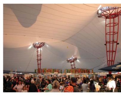
As shelters for performance stages they can provide a proscenium-like setting without the heavy structure required with other materials. Their ability to provide vast clear span space assures clear sight lines for the audience with minimum of supporting posts. These attributes enable a designer to use his imagination to the fullest.
