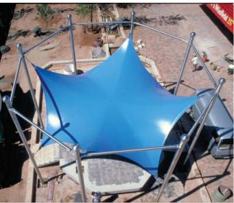
Prestressed membranes such as tension membranes or air-supported structures. Tension membrane structures assume double negative (anticlastic) curvature. Air supported structures assume a double positive (synclastic) curvature.
