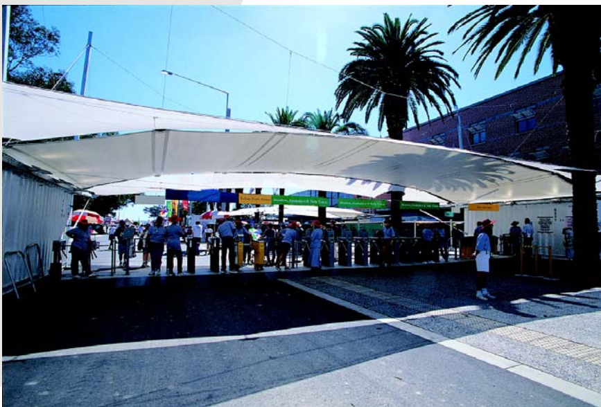
RAS Temporary Entry Structure, Sydney Showgrounds (Award of Excellence - Small Structures Category, LSAA Design Awards)
