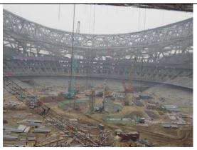
Main Stadium - or Birdnest Stadium has most steelwork completed and installation of both roof transparent ETFE membrane and lower PTFE/Glass acoustic liner currently underway. ETFE membrane contractor - Covertex GmbH. PTFE/Glass membrane contractor - N&L China
