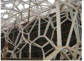
Swimming Complex or WaterCube - work on double layer ETFE cushions currently in progress. ETFE membrane contractor - Vector Foiltec
