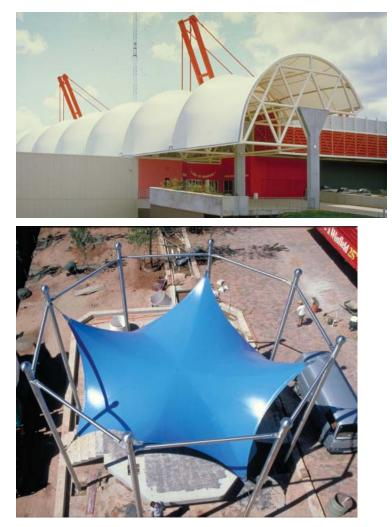
Non prestressed membranes such as tents, sails and air (or other medium) filled structures, which are originally slack in the unloaded condition and assume shapes of either single or double curvature when loaded.
