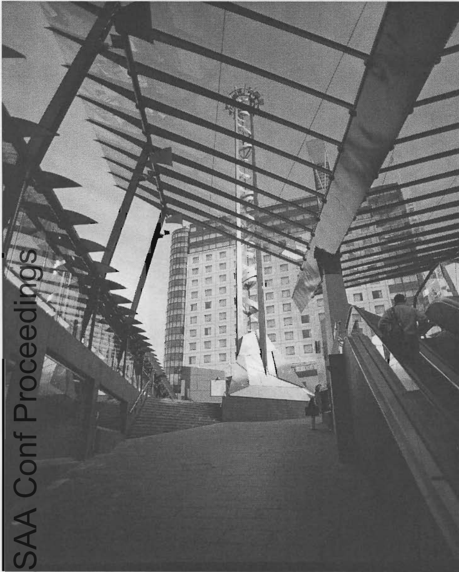
Figure 13: Completed Canopy Structure
