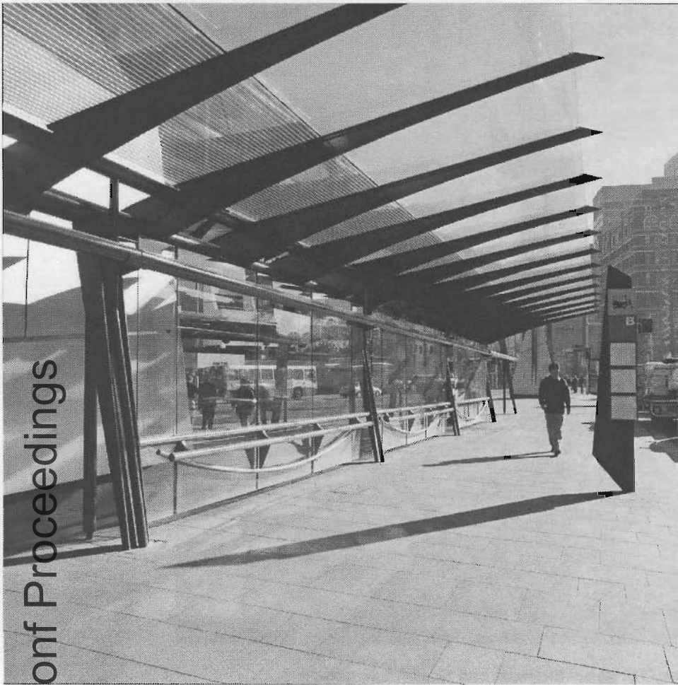
Figure 15: Details of Slender Cantilever Blades
