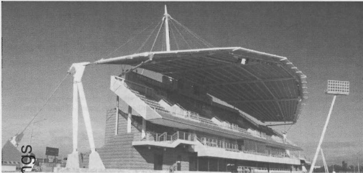
Figure 1. Grandstand Roof of Hockey Centre
