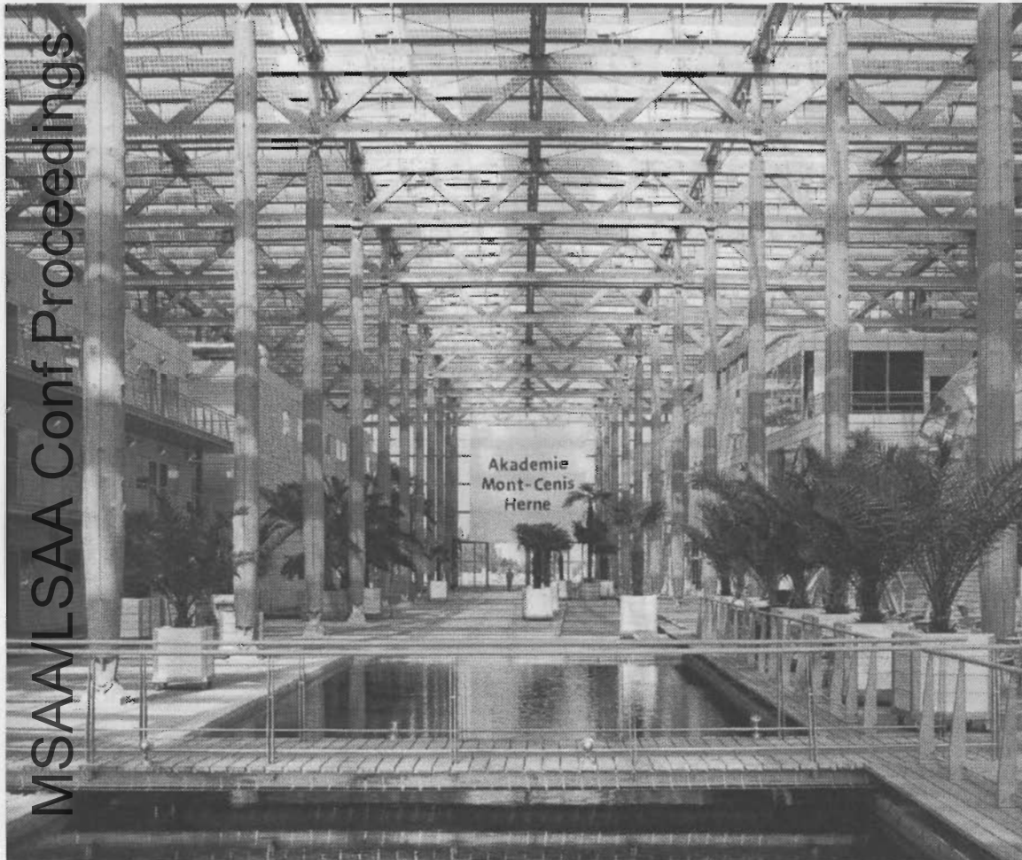
Fig 1. Training Centre in the Ruhr. Interior with classrooms and offices as separate buildings under an external skin
