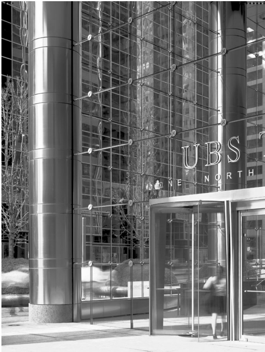
Figure 6. One North Wacker Drive End Bay with Portal
