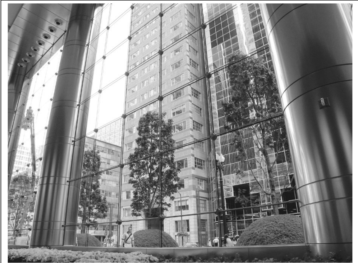
Figure 5. One North Wacker Drive Interior View
