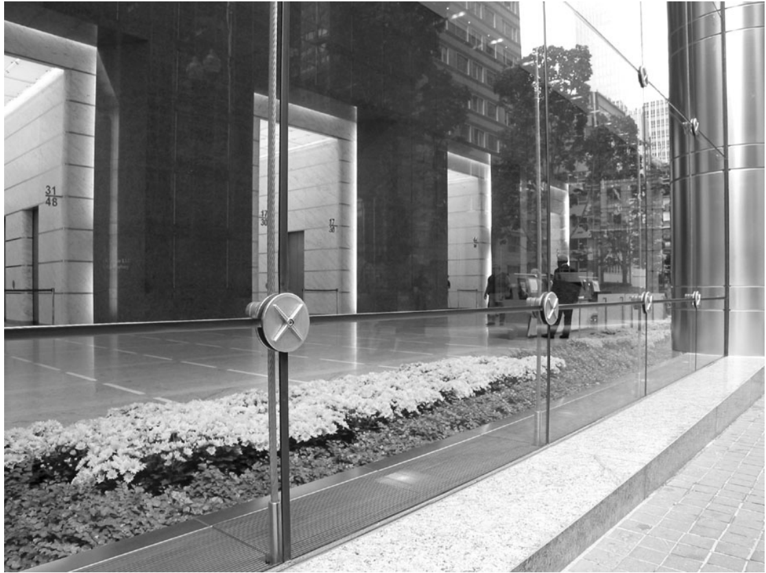
Figure 3. One North Wacker Drive Exterior View
