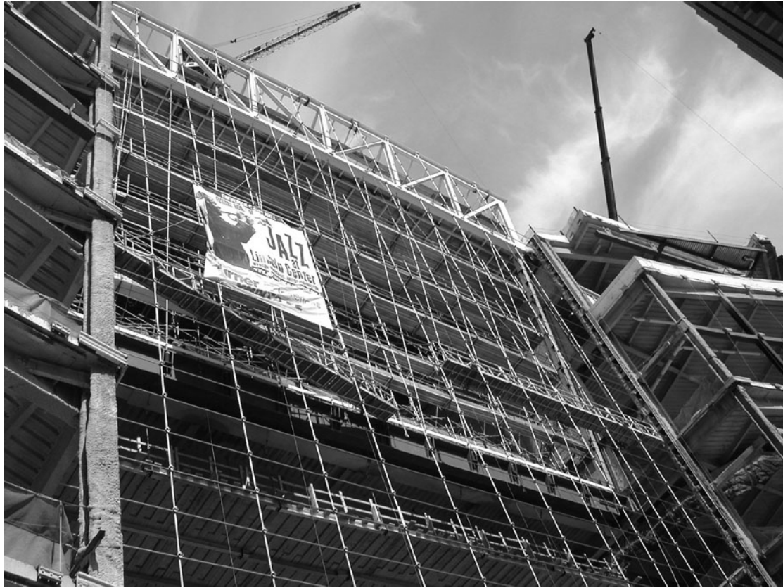
Figure 8. AOL Exterior View
