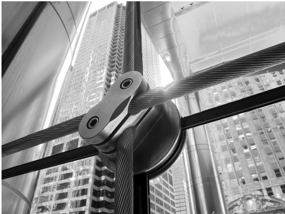
Figure 2. One North Wacker Drive Node Detail
