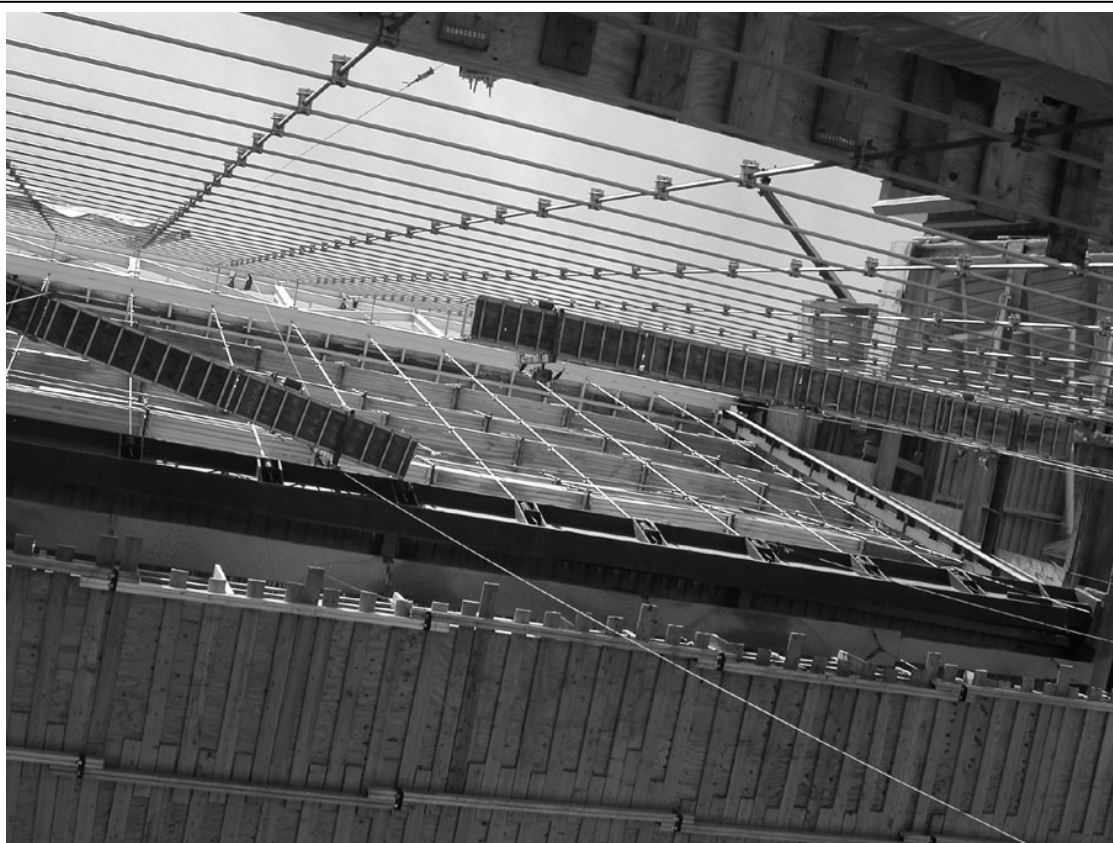
Figure 9. AOL Interior View
