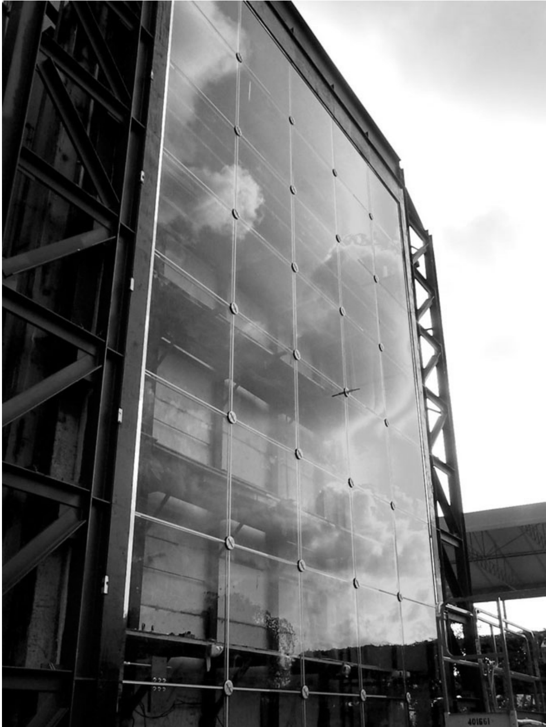
Figure 7. One North Wacker Drive Mock-Up Test
