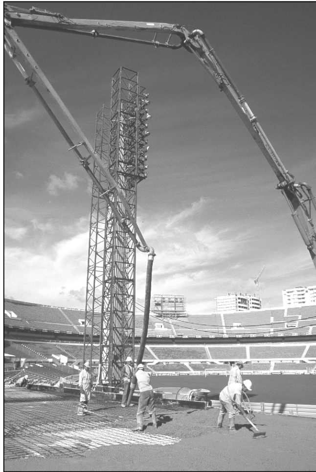
Figure 3: Work on new stadium proceeding with existing stadium in background
