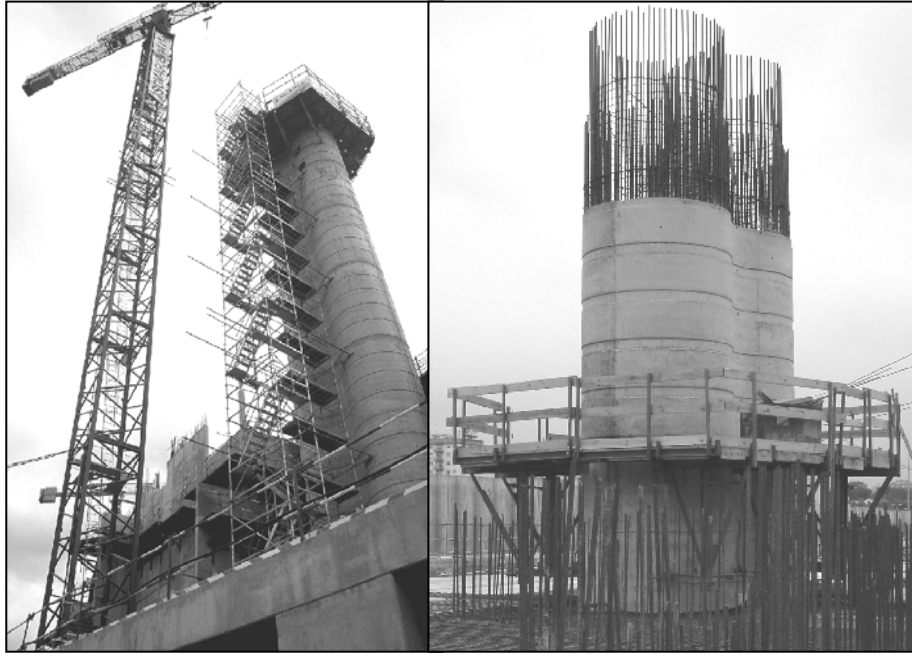
Figure 6: Supercolumn under construction
