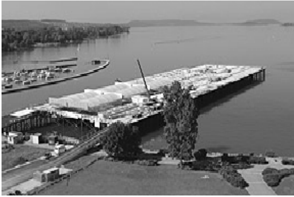
Pier under construction
