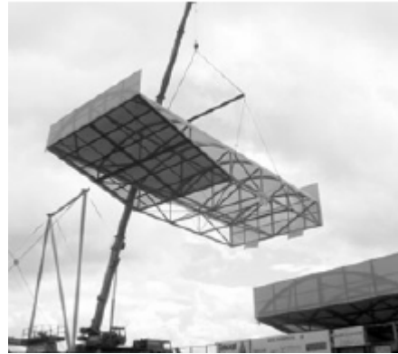
Lightweight elements lifted into place
