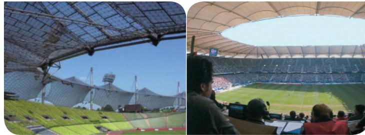
Frei Otto's German Pavilion at Expo 67 was the fore runner to his famous Munich Olympic Stadiums. Many large modern stadia have been built using a cable structure supporting, and giving form to tensioned fabric roof panels. With a complete stadium, the inner opening has a large tension ring made from cables. The radial cables are tensioned and resisted by an outer compression ring which in turn is supported by many outer columns. Connections and cable end fittings are a vital part of the design.
