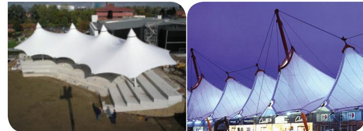
The main design loadings are the initial prestress in the fabric and wind loads - dead weight is very small. Prestress is generated by patterning the fabric from standard width rolls to be a smaller size. The fabric is stretched to its supporting system by adjusting the length of edge cables, tensioning of side guys, jacking up of internal masts or a combination of methods.
