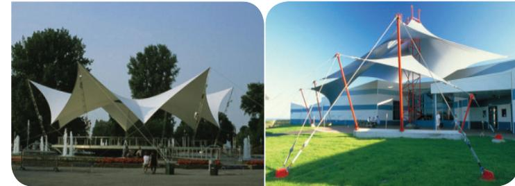
To obtain the curvatures, major support elements such as masts and arches are used. Fabric materials include teflon or silicon coated glass, PVC coated Polyesters, foils and shade cloth.
